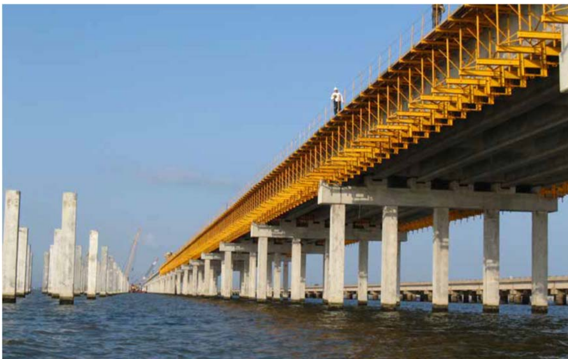
Photo 7.1 I-10 Twin Span Bridge New Orleans & Slidell Reconstruction after Hurricane Katrina
