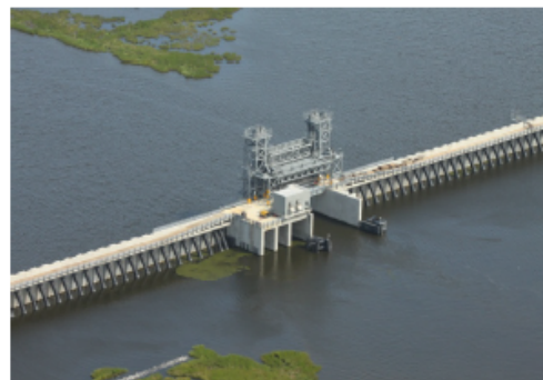
Vertical Lift Gate at Bayou Bienvenue
