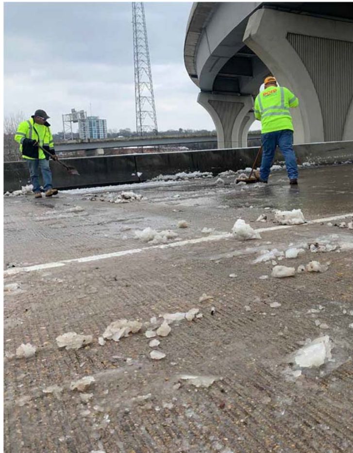
Photo 7-2 Removing ice on a ramp at the Shreveport I-20/I-49 interchange 2021
